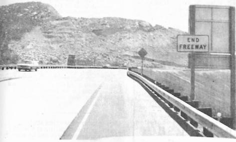
Here is upper end of 35-mile completed I-8 from SD to Deadmans Curve, fast disappearing is mountain ahead. At top the bank is taking shape, will be cleared to grade of paving when lanes will go nearly straight ahead, eliminating dangerous curve.
